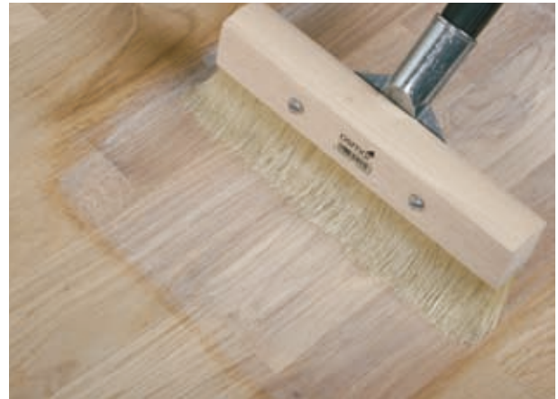
4) Applying Osmo Hardwax-Oil White Foundation 3040 with a Floor Brush
